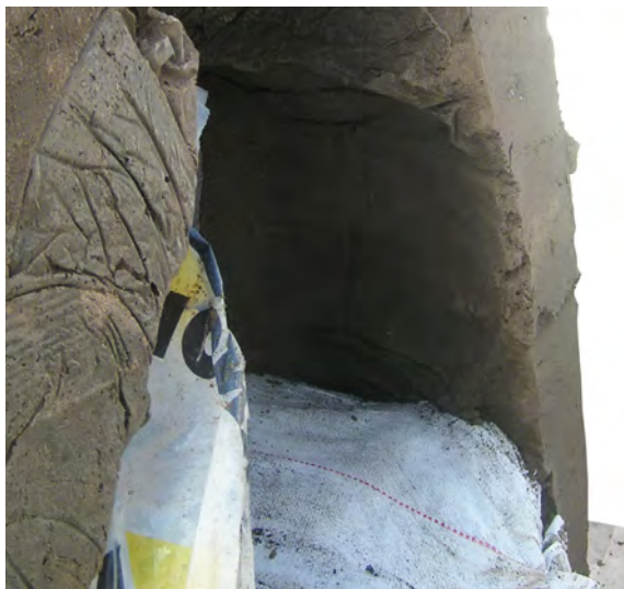
Fig. 213. Step 5. Removing other sandbags without opening them
