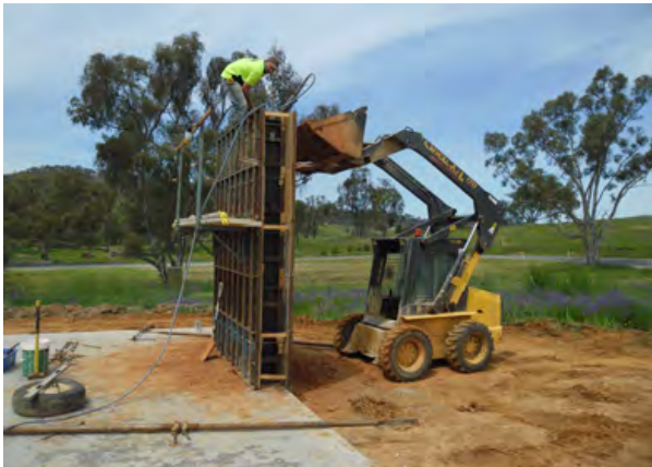
Fig. 106. Soil delivery
