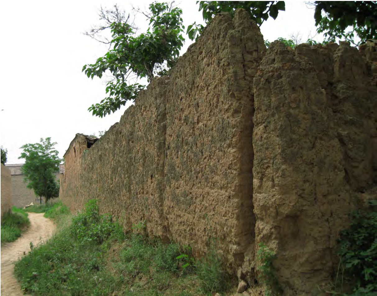
Fig. 60. Eroded rammed earth wall in China
