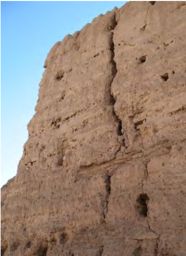
Fig. 90. Consequences of major shrinkage
