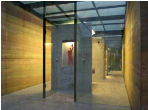
Fig. 171. Glass roof system in relation with earth walls
