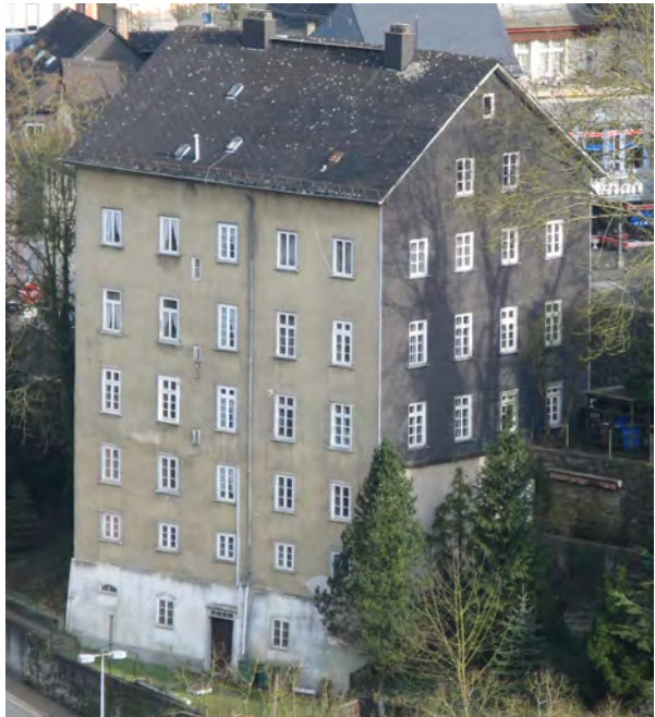
Fig. 32. Rammed earth building in Weilburg, Germany (1826)
