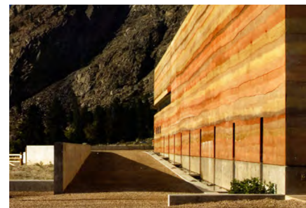
Fig. 68. Protective concrete footing
