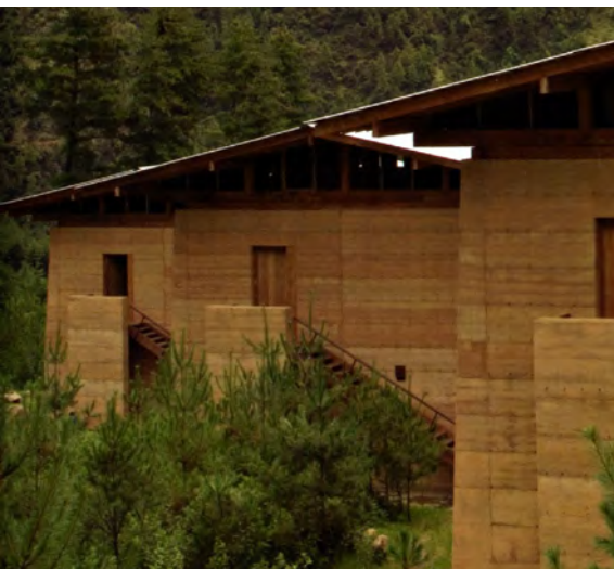
Fig. 49. Differentiated wall thickness. Housing in Bhutan (2005)
