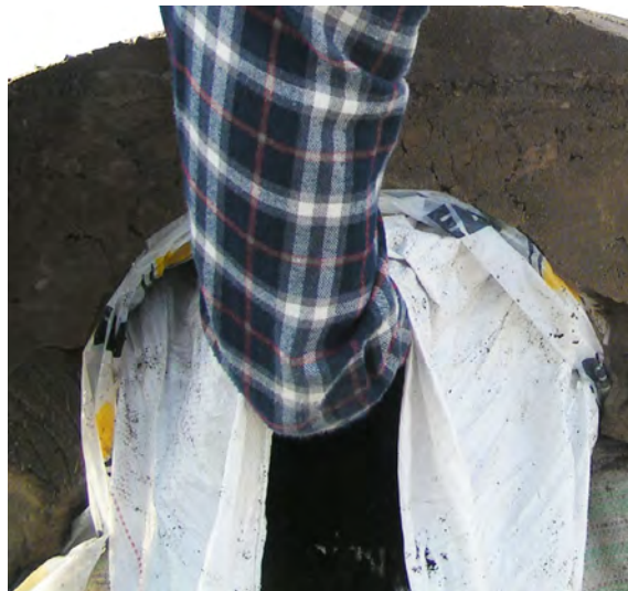
Fig. 212. Opening top sandbag and removing sand
