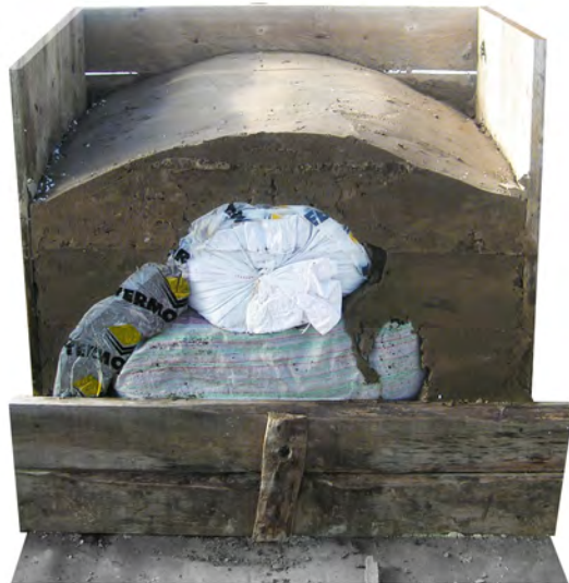
Fig. 211. Step 3. Pouring light concrete and removing formwork
