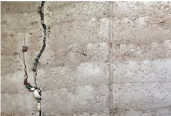
Fig. 93. Typical rammed earth shrinkage crack
