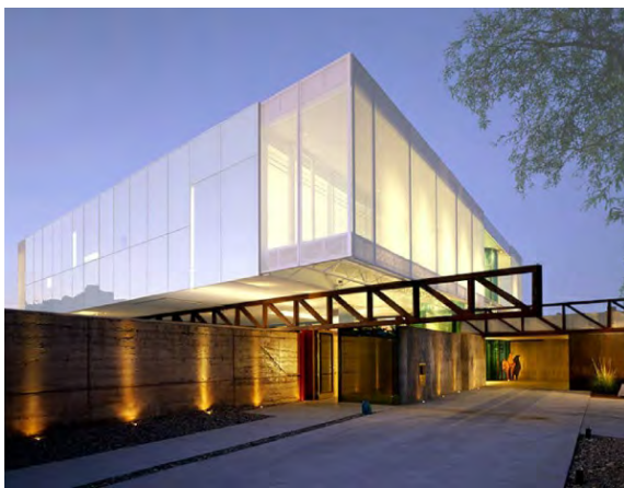
Fig. 170. Loadbearing steel beam in relation with earth wall
