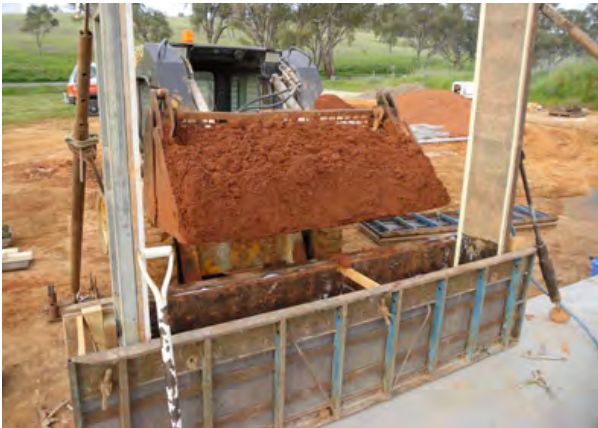
Fig. 105. Soil delivery
