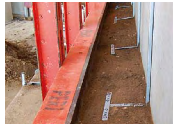
Fig. 99. Sliding anchorage to supportive concrete wall
