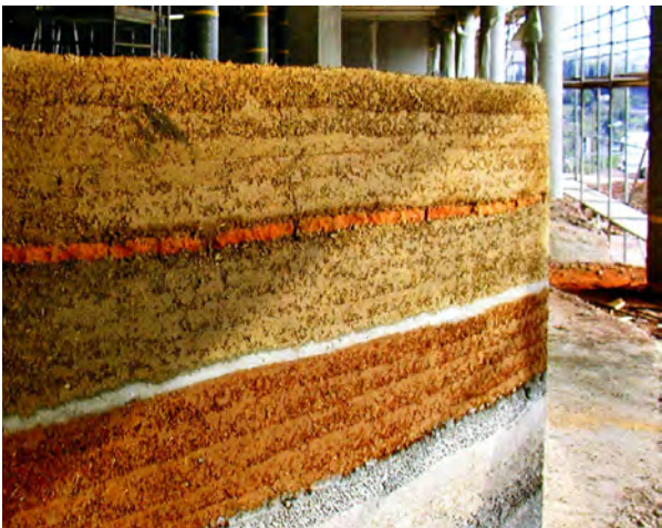
Fig. 80. Mixture of straw loam and expanded glass
