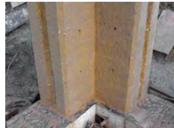
Fig. 95. Corner element with tongue-in-groove joints
