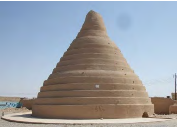
Fig. 46. Ice storage made of mud brick in Iran
