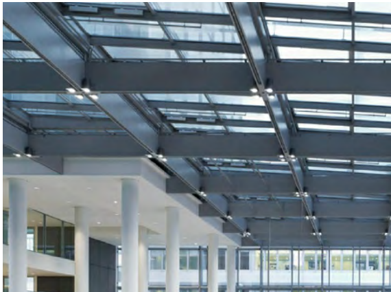
Fig. 169. Beams with integrated ventilation (Licht Kunst Licht)
