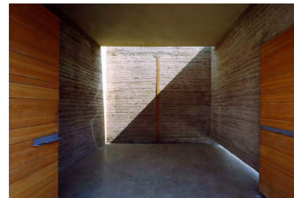
Fig. 70., 71. Uplifted rammed earth wall on a metal beam with double anchorage. Chapel of rest in Vorarlberg, Austria (2001)
