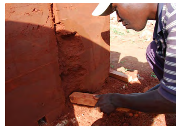
Fig. 101. Repairing rammed earth element
