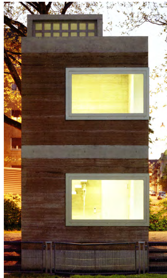
Fig. 41. Concrete bond beams. Chronometry Tower, Zurich
