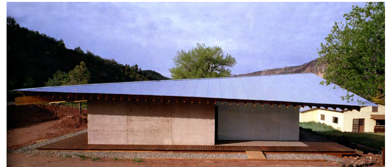
Fig. 72. Moisture protection by overhanging roof. Center of Gravity Foundation Hall in Jemez Springs, New Mexico (2003)
