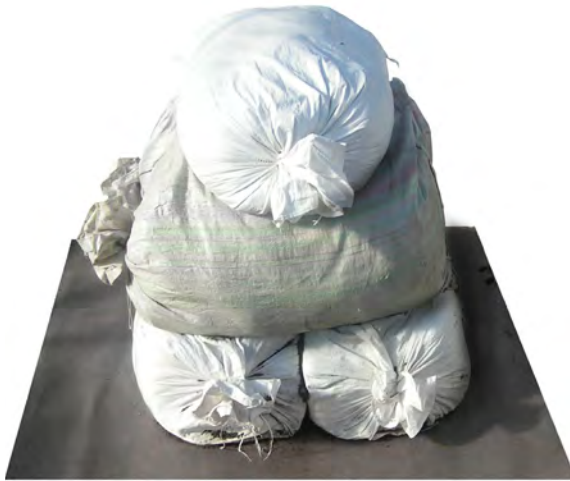
Fig. 209. Step 1. Placing sandbags
