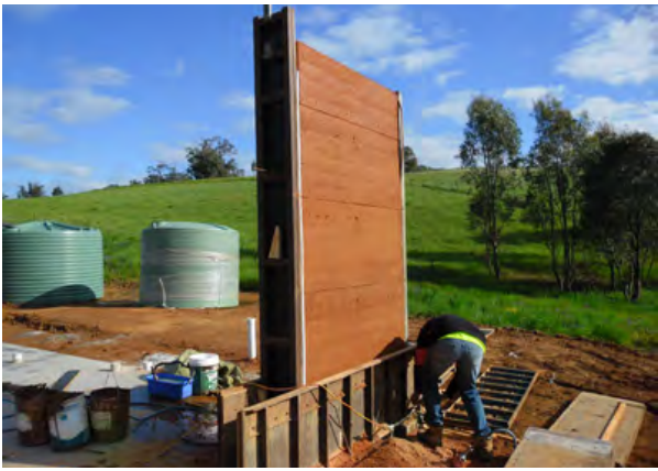
Fig. 109. Removing formwork
