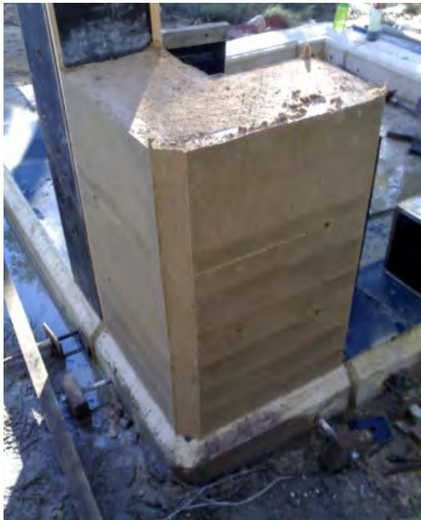
Fig. 53. Preferable angle construction method
