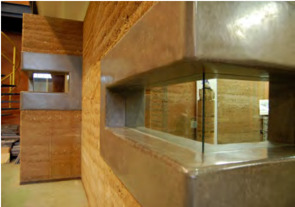
Fig. 39., 40. Rammed earth wall with corner window by "LEEMWERK"
