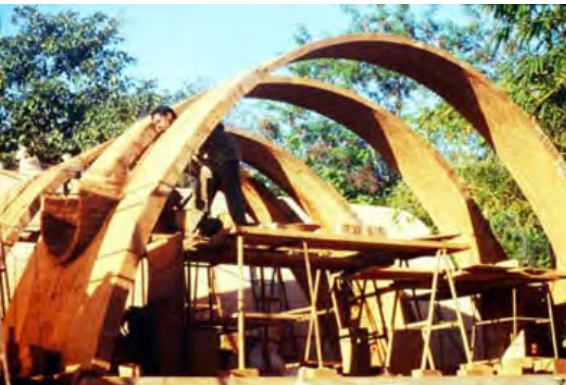
Fig. 48. Vaults of compressed earth blocks by Nubian masters
