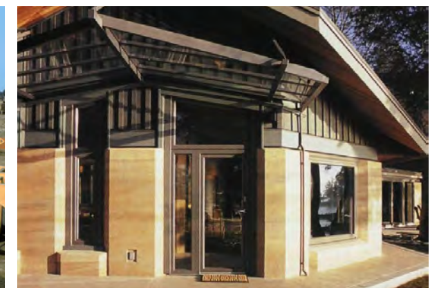
Fig. 67. Earth walls covered with transparent acrylic water repellent
