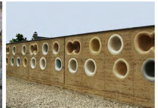
Fig. 96. Control joint for graveyard wall in Spijk by “LEEMWERK”
