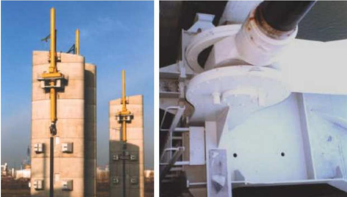
Fig. 9.5: Hartel Canal Barrier – global view of projected cylinders and detail of the cylinder joint to one of the gates [19]
