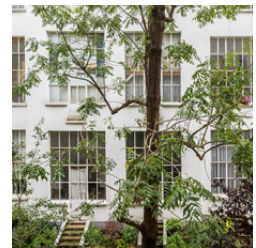
The atelier facade
