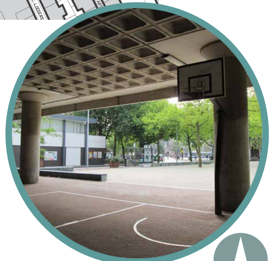
Open ground floor below the parking garage, overlooking the square
