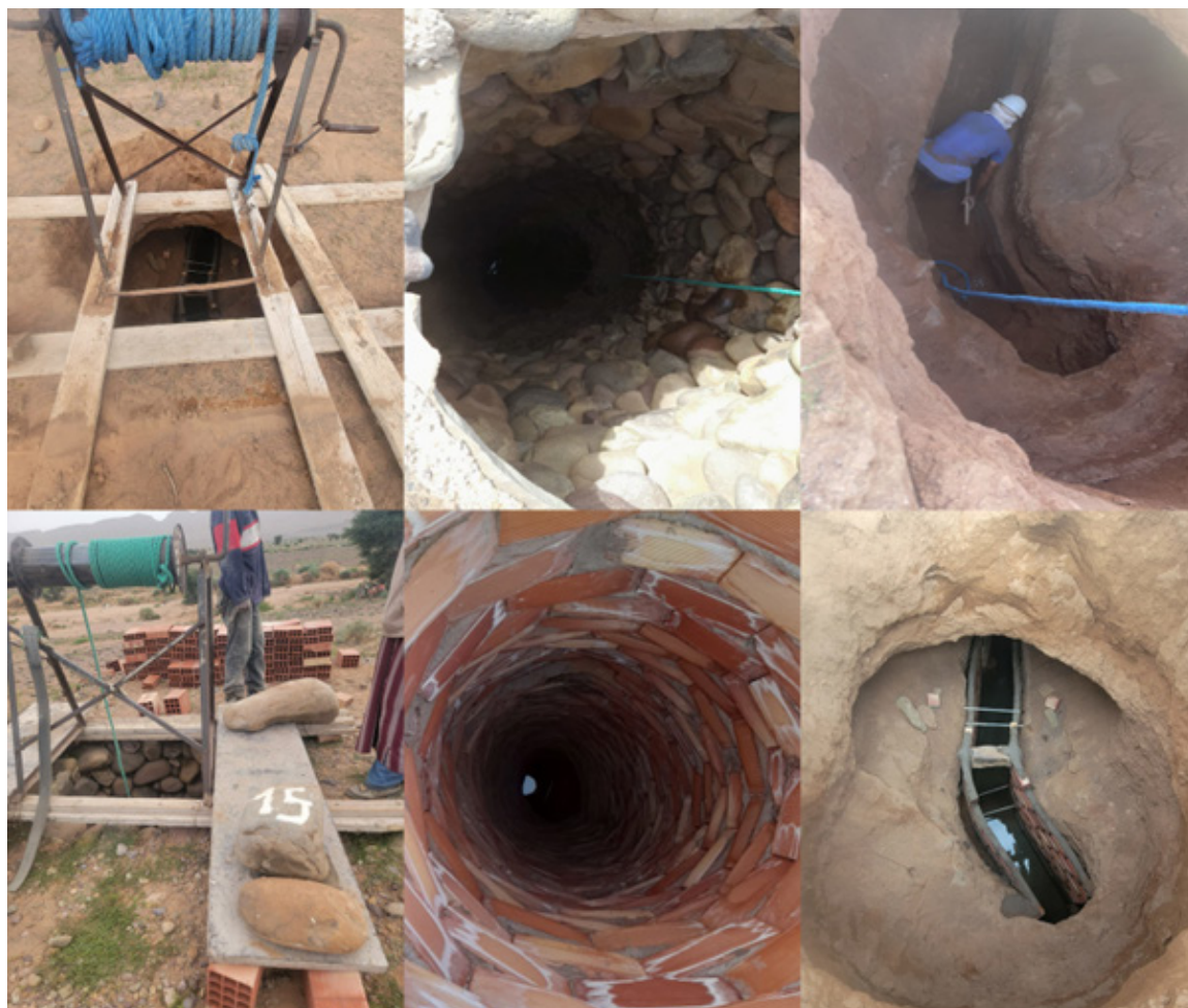
^ Fig. 4 Example of recent maintenance of a khattara near Ait Zeggane (Morocco) with modern techniques and materials. On the left you can see the systems for moving the material along the wells, in the center you can see two wells renovated with stone and bricks respectively, on the right you can see the maintenance work, during and after in a slightly kilned well (Source: Mhammad Houssni, 2024).
