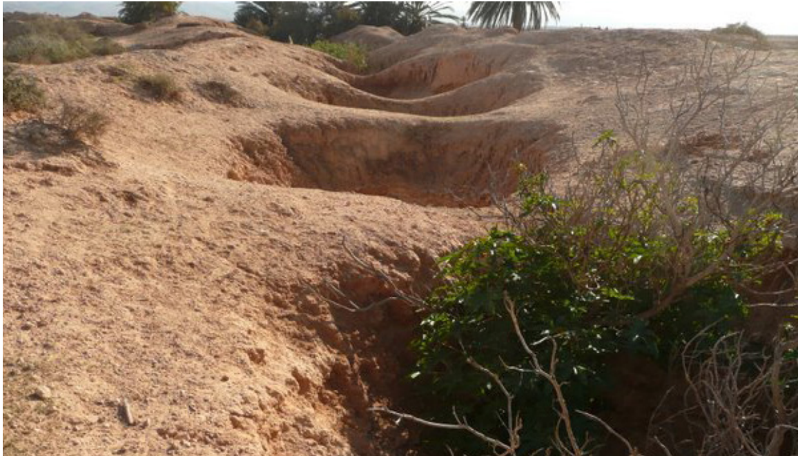
^ Fig. 4 The tops of khattara maintenance shafts with signs of dereliction and overgrown vegetation, threatening their collapse, Guelmim region, Morocco (Source: Cristiana Strava, 2010).
