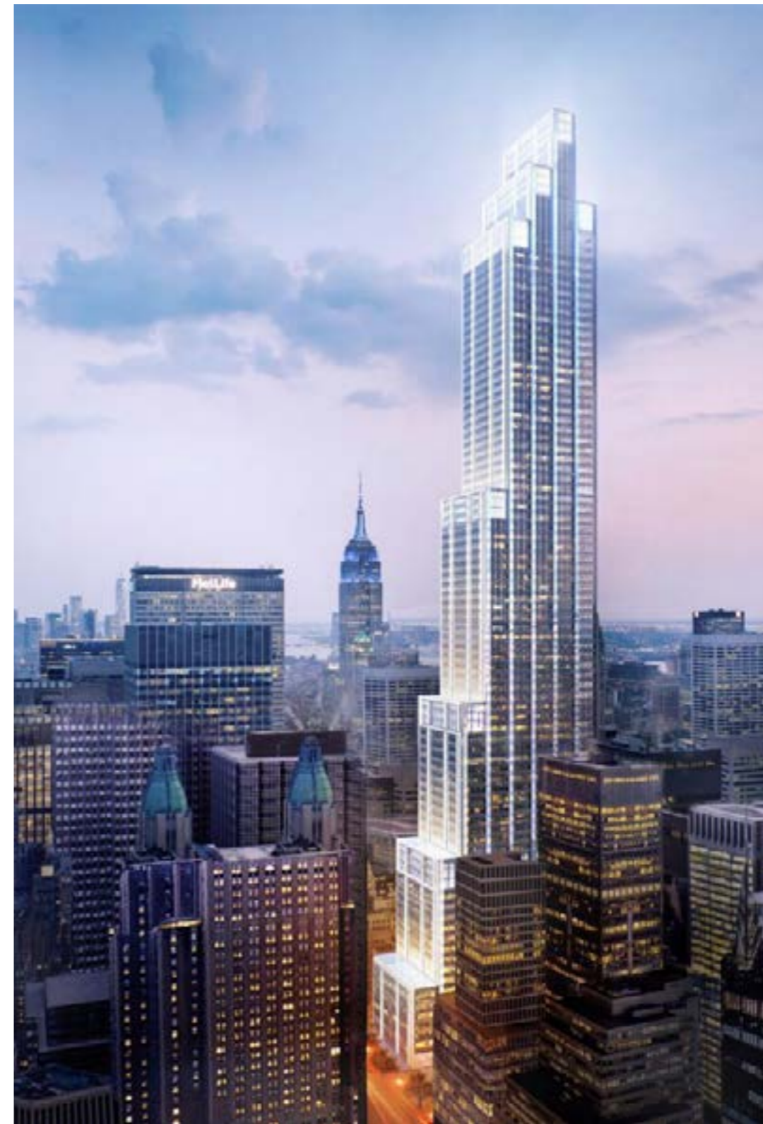
New JP Morgan Chase Headquarters In Construction
