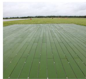
Figure 9.4: Assembled Temporary Runway [44]
