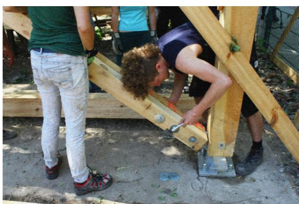
*The structure was built using traditional carpentry methods, without large machinery. Pine wood, threaded rods, bolts, and Geka dowels secure the elements, allowing for easy assembly and disassembly.*
