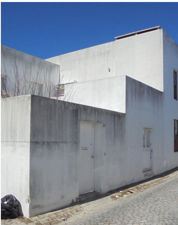
Figure 4: An example where the panel of the gate is white not creating contrasts in the façade. (Source: Authors)
