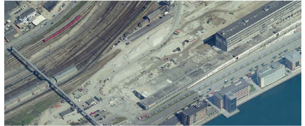
Derelict space at the ring road
