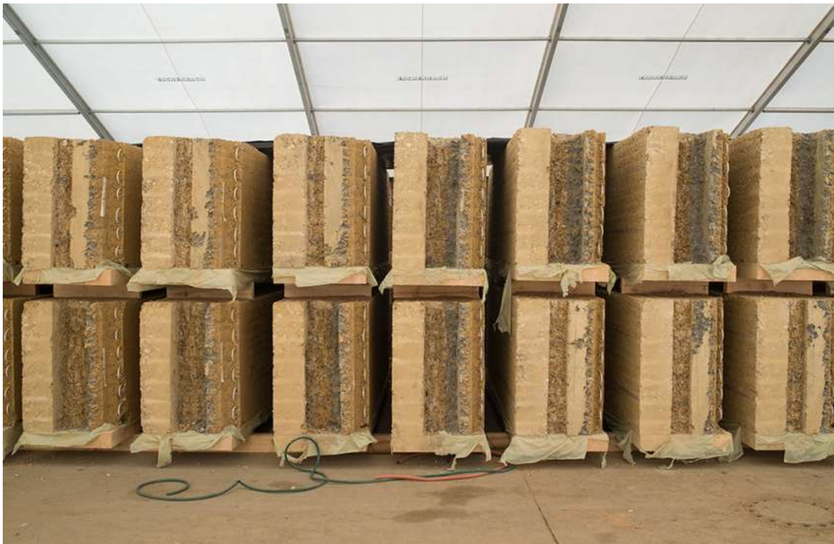
Figure 3.2. Rammed earth on-site prefabricated rammed earth wall panels.
