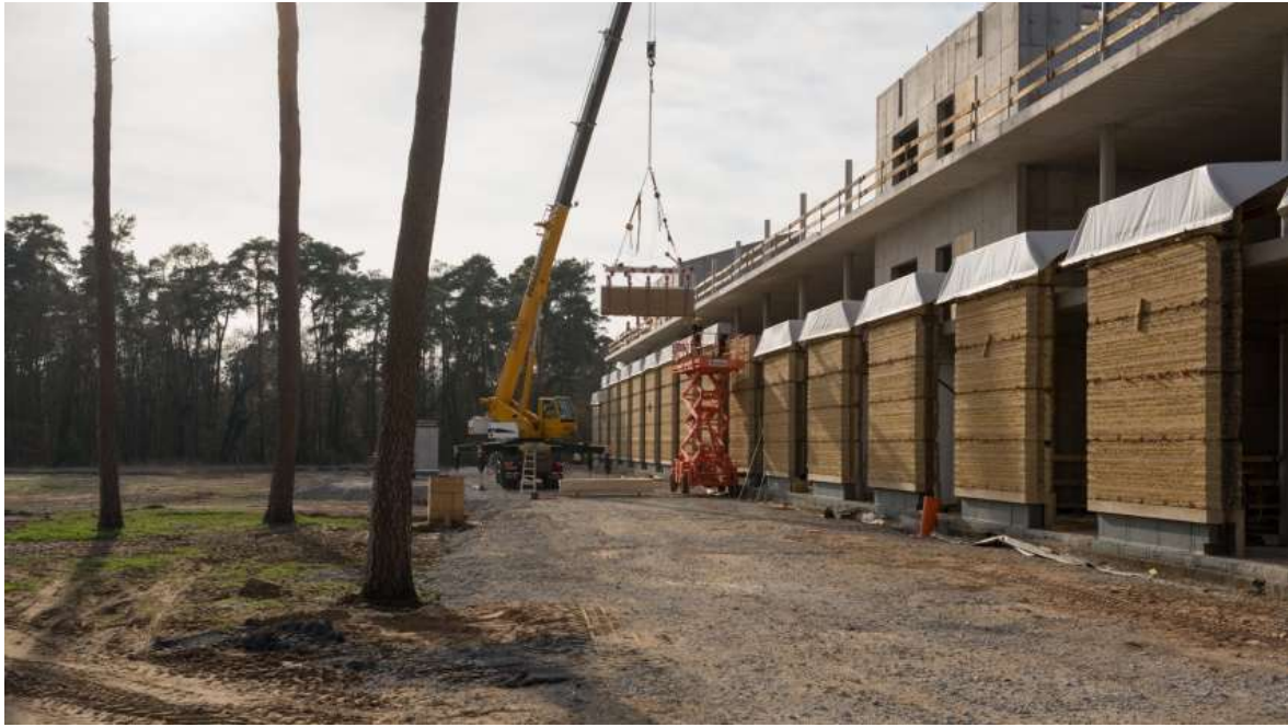
Figure 2.11. Prefabricated rammed earth panel being craned into place on the Alnatura Campus project.
