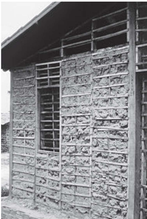
Figure 2.15. Prefabricated wattle and daub system in Brazil.
