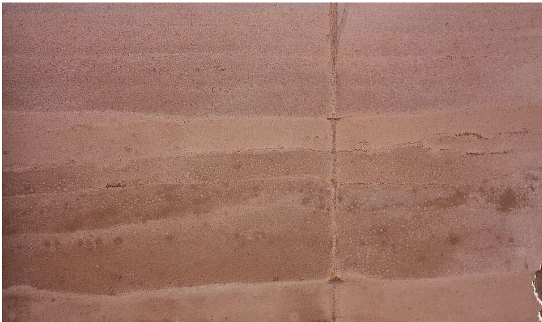
Figure 2.10. Rammed earth wall surface.
