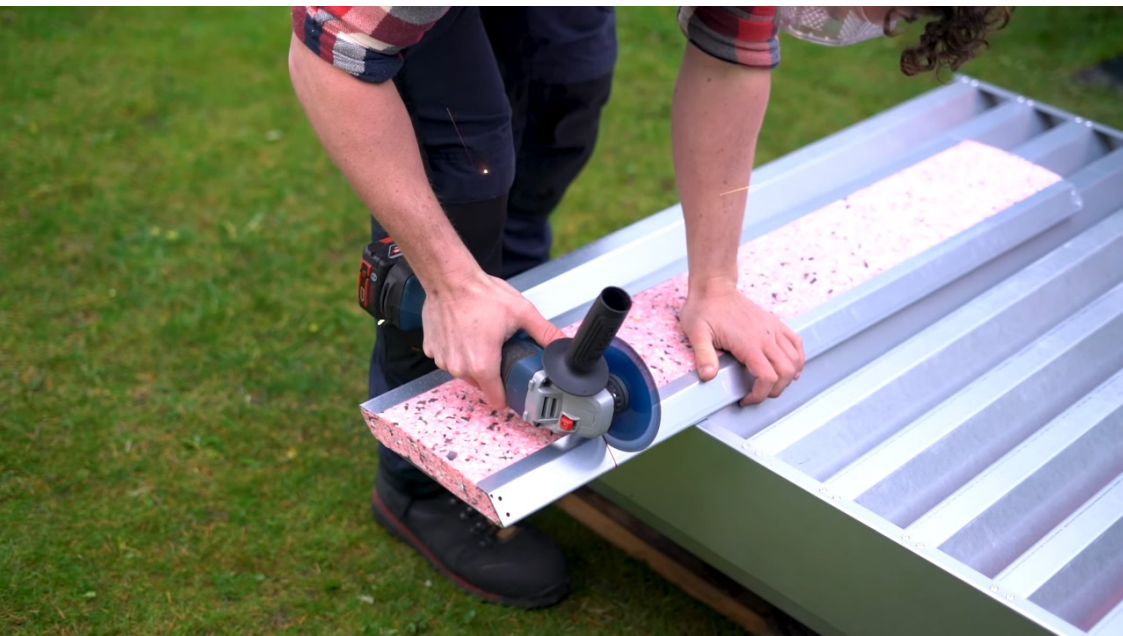
Figure 17: If a cable hole is needed, a drill, angle grinder and rivet gun are required to install the cover of Reducd
