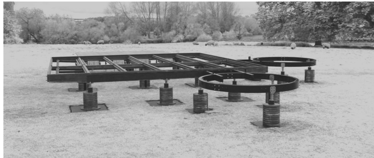
figure 8. Jean Prouvé prefab shelter, assembled base with metal anchors (Wallpaper* magazine, 2015)
