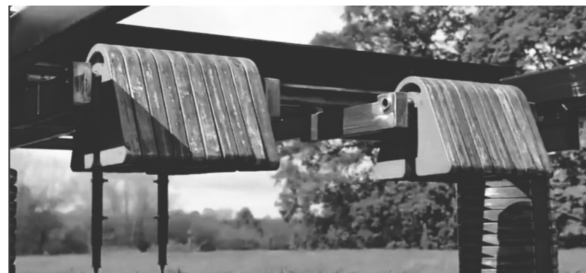
figure 8. Jean Prouvé prefab shelter, assembled base with metal anchors (Wallpaper* magazine, 2015)
