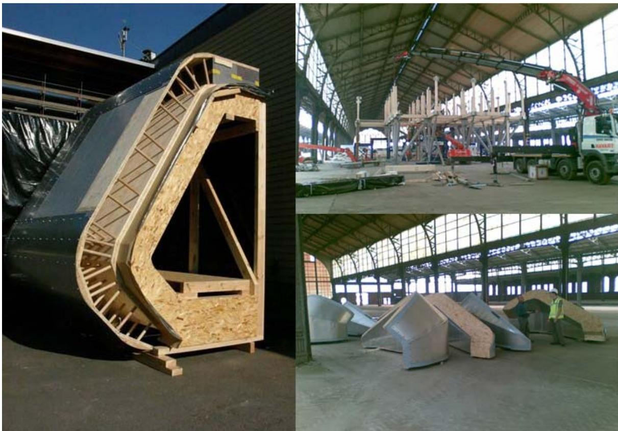
Figure 56: Final building modules [Source: IPF]
