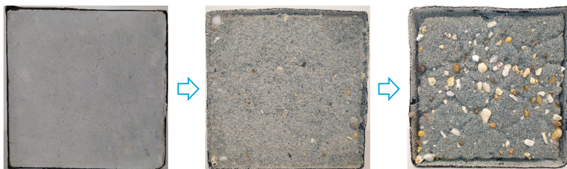
Figure 2.1.2 Surface condition evolution of an AASC with severe surface scaling damage due to freeze-thaw cycles.
