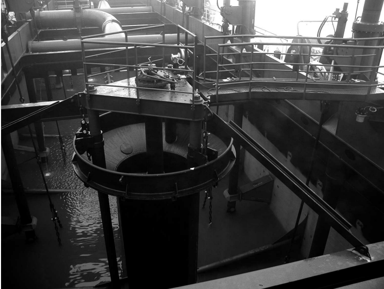
Figure 2.6: Overflow weir.
