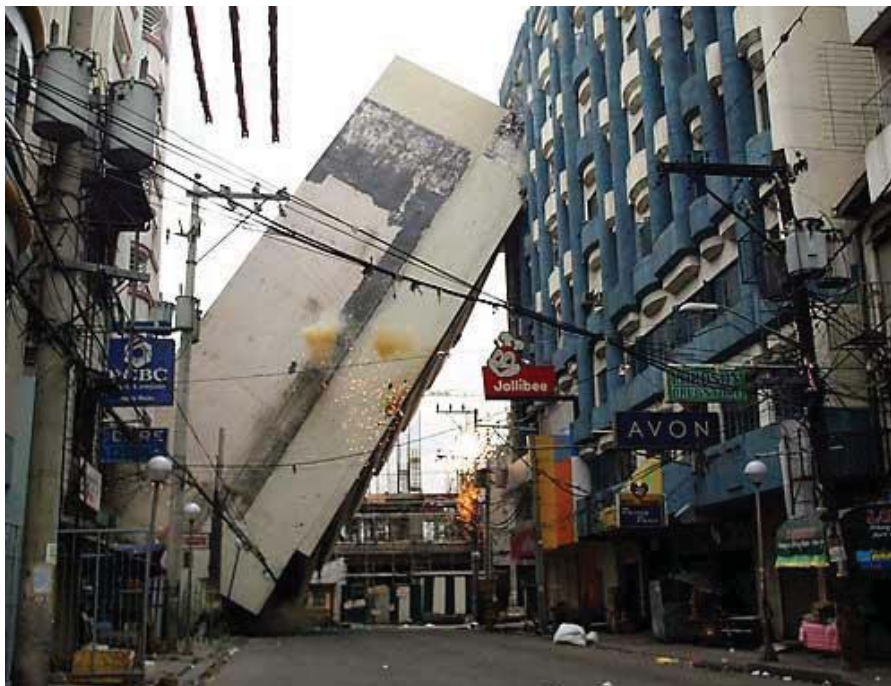
Figure.3.3 Domino type collapse; Overturning office building in Manila impacting adjacent apartment building [Source: http://www.archidose.org ]
