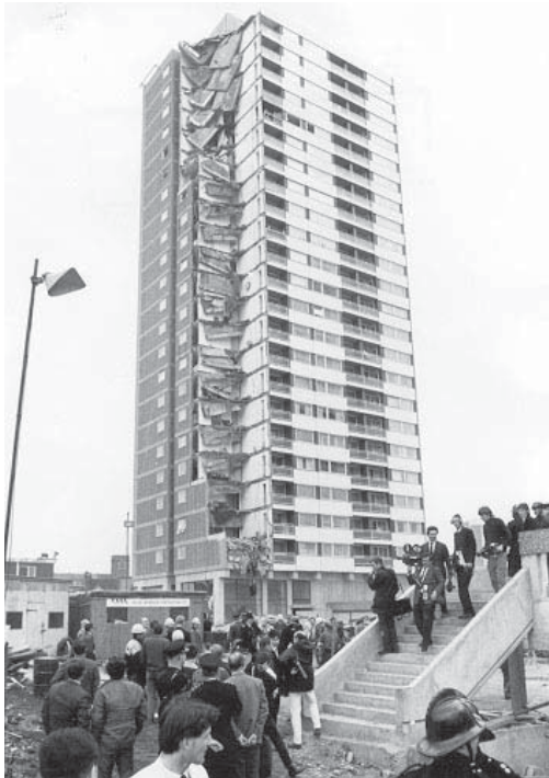
Figure.1.1 Collapse of Ronan Point
