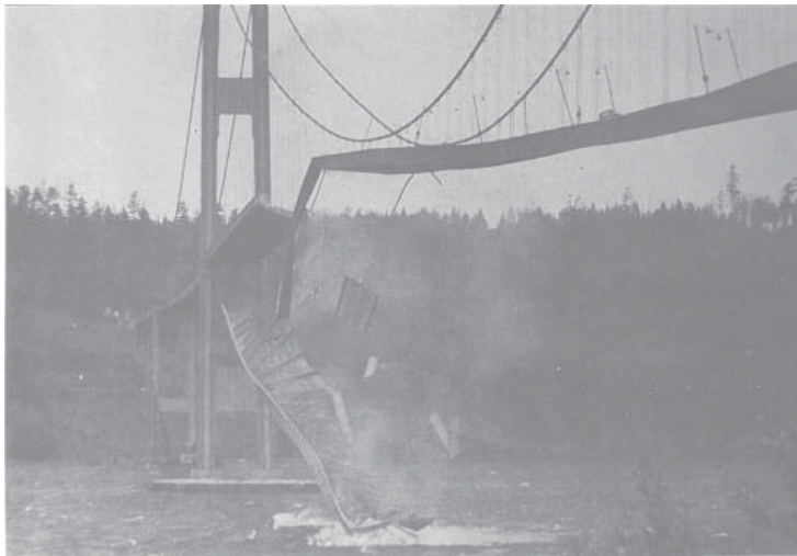
Figure.3.2 Zipper type collapse; Tacoma Narrows Bridge [Source: http://www.jalopnik.com ]
