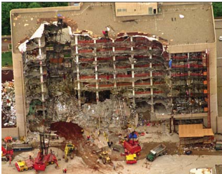
Figure.3.6 Murrah Federal Building after the bombing in 1995 [Source: http://www.911review.com ]
