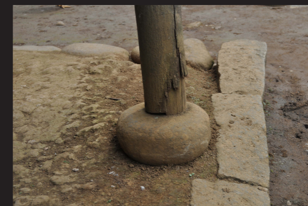
FIG. 14-18 (LEFT TO RIGHT CLOCKWISE, 2017) 14. A SMALL HOME, FIRE WOOD AND CHICKEN CAGES STOCKED UNDERNEATH 15. REED AND PALM LEAVES AND FIBRES AS ROOF CLADDING 16. BAMBOO AND WOOD WINDOW HATCH 17. INTERIOR OF A BIG HOUSE, WOODEN FLOOR, PLAITED BAMBOO WALLS 18. WOODEN BRANCH AS COLUMN, HELD IN PLACE ON RIVER STONE BY PRESSURE FIG. 19. (PREVIOUS PAGE) DRAWING OF HOUSE + FLOOR AND FOUNDATION ELEMENTS
