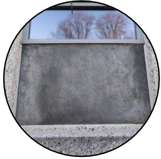
Reused stone panel
