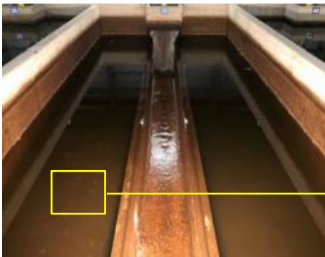
Figure 97a Full-scale RSF during ETSW 5 m/h up-flow
