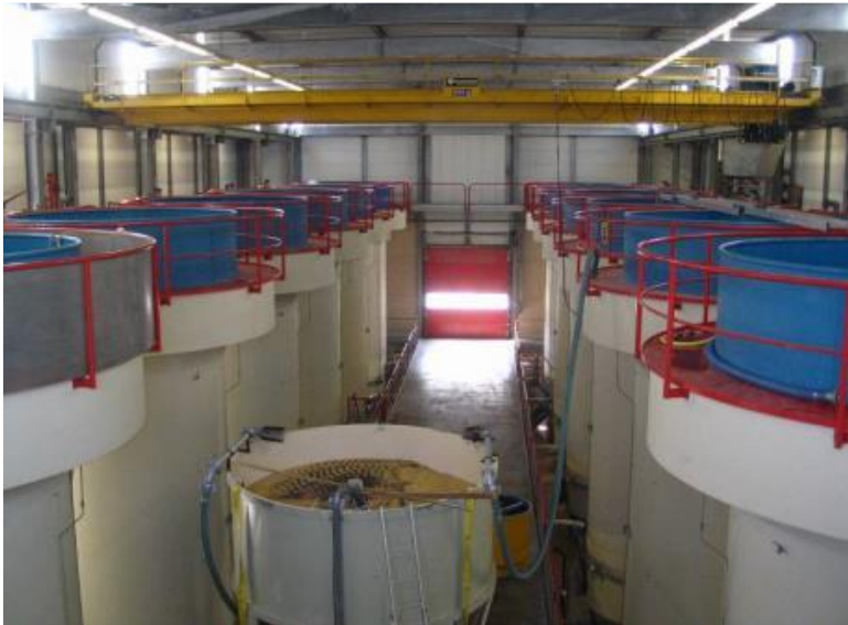
Figure 65 Full-scale pellet-softening reactors located at Waternet (Amsterdam, the Netherlands). The unit consists of 12 Amsterdam reactors with reactor diameter D = 3.0 m (van der Veen and Graveland, 1988).
