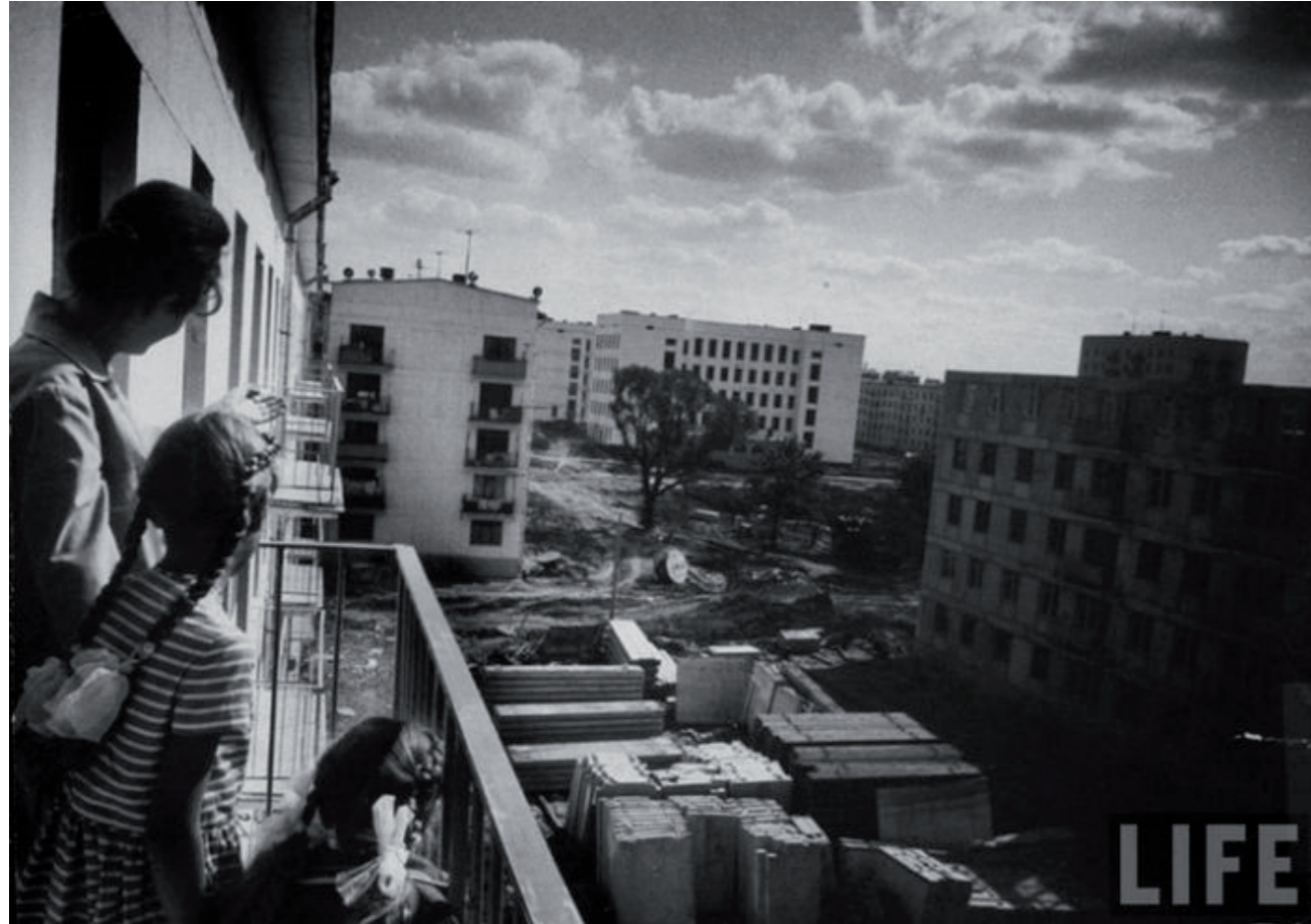
Construction of „Khrushchovka“ - first residents
