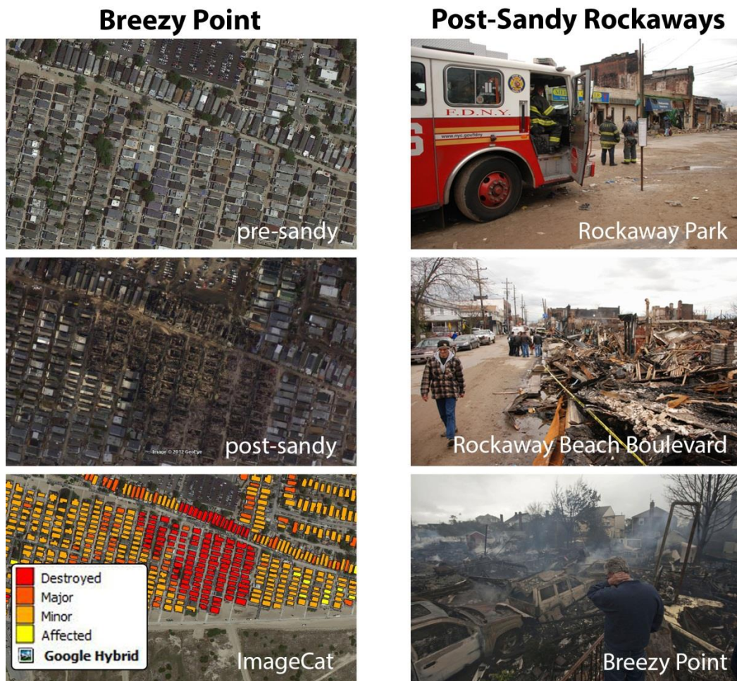
Figure 2-22 - Short-circuit fires burned down complete neighbourhood at Breezy Point and some other places in the area (Photographs by USACE and Nathan Kensinger amongst others)
