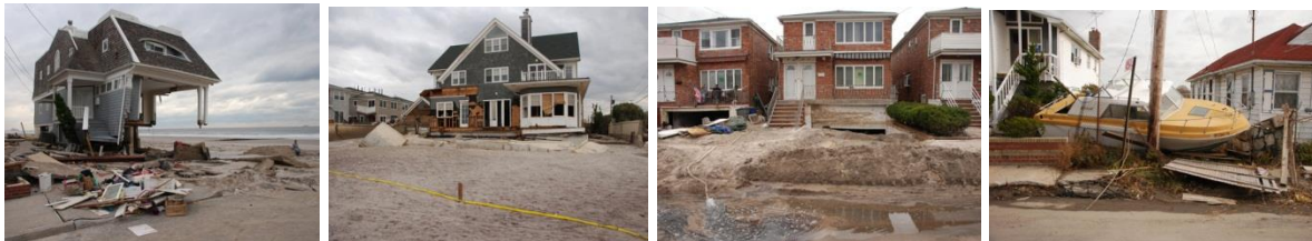
Figure 2-20 - The oceanfront of The Rockaways has been almost completely demolished by wave battering (photos by Nathan Kensinger)
