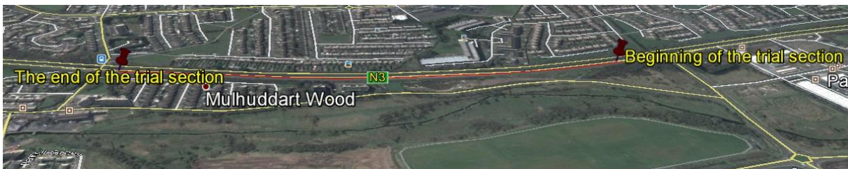
Figure 3. Satellite image of the trial road section
