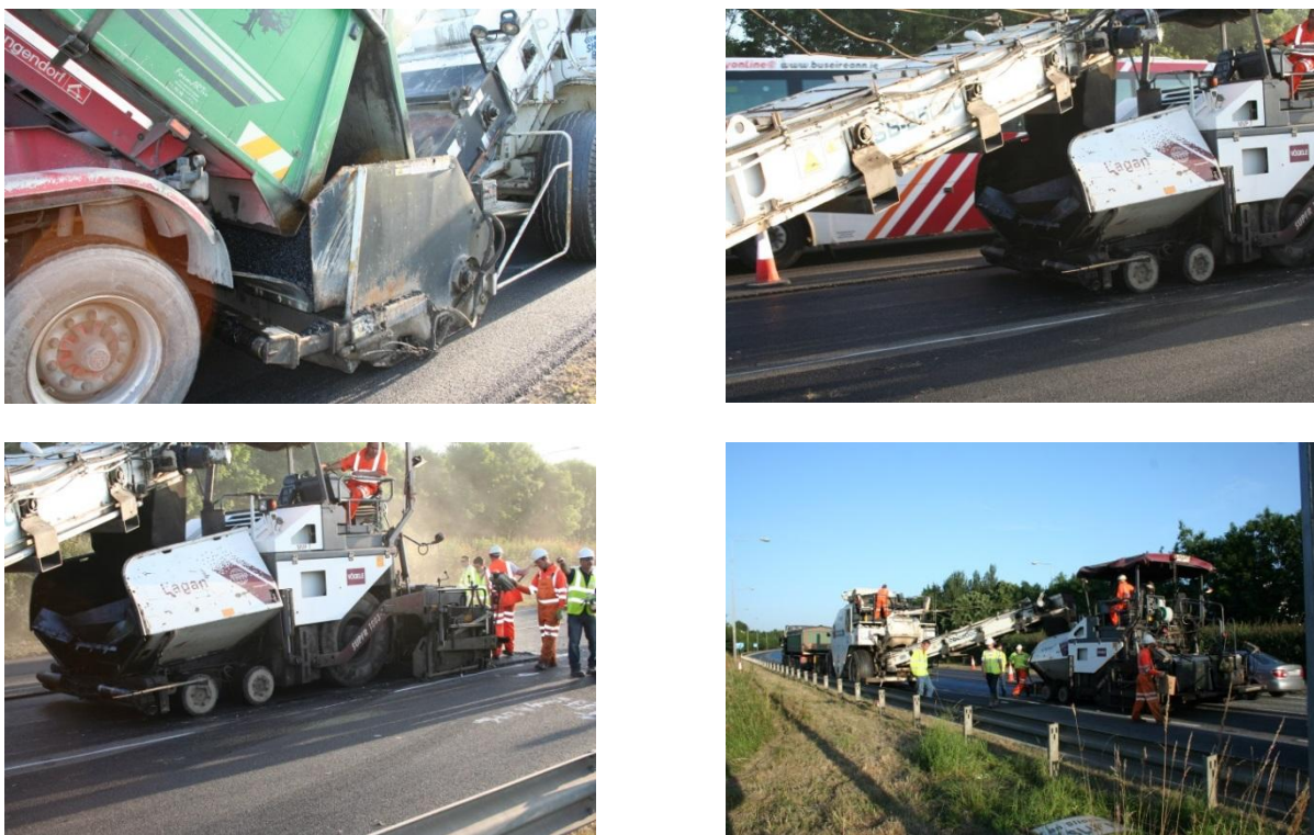
Figure 5. Paving process of the trial section
