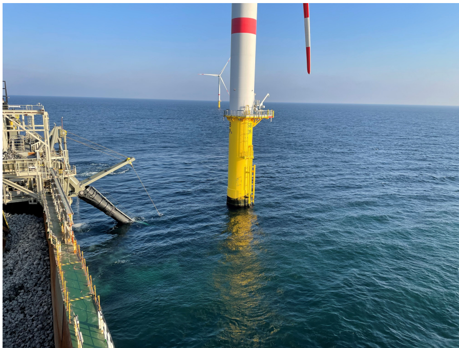
Figure 1.1: IFP of the Rockpiper, depositing rock next to a monopile. [29]
