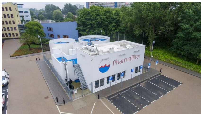
Figure 15: The Pharmafilter installation on the premises of Reinier de Graaf Hospital. The system is currently in partial operation, focusing on wastewater treatment to remove pharmaceutical residues and other contaminants, with the treated water being reused within the hospital.
