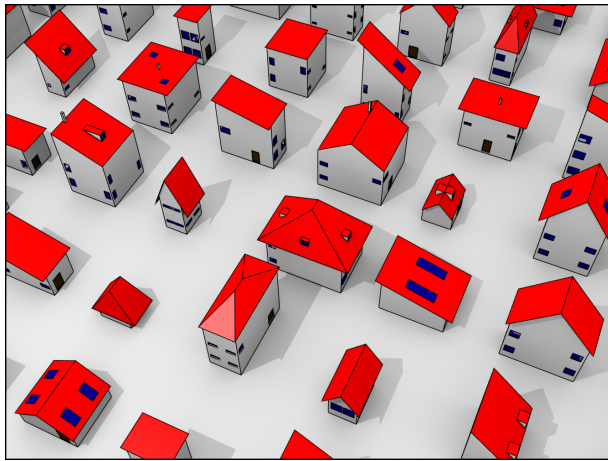
Figure 4: Visualisation of a small spatial extent of the LOD3 dataset that is a semantically enriched boundary representation. The colours represent the different semantic classes.
