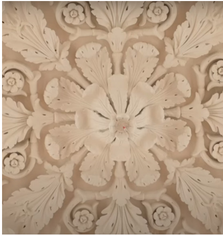
Figure 14: The hidden smoke detector in the middle of the ornamentation (State Library Victoria, 2020).
