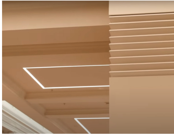
Figure 15: The hidden ventilation shafts, seen on the right hand side of the image and the sound absorbing panels, seen on the left hand side outlined by the light (State Library Victoria, 2020).
