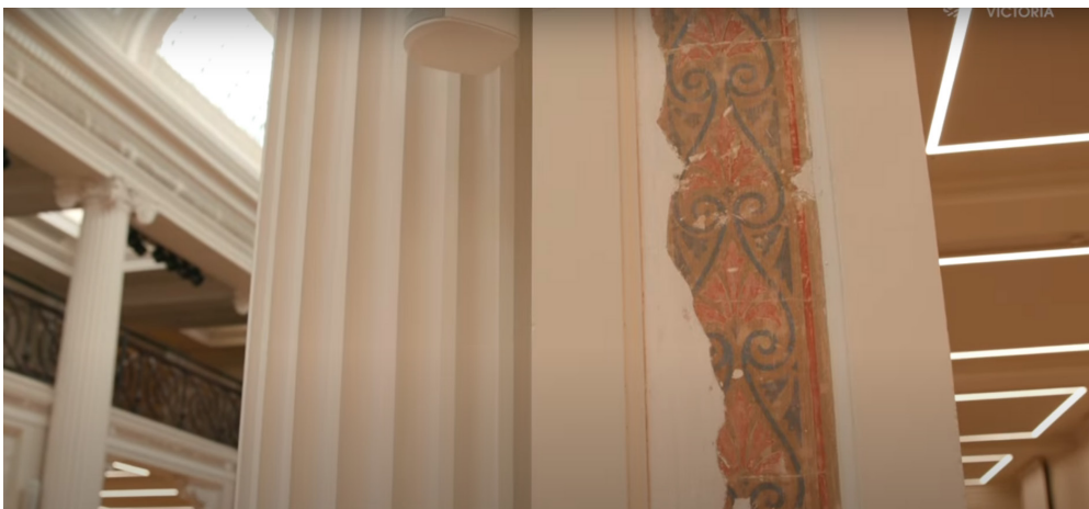
Figure 13: The original wall decoration uncovered after removing the multiple layers of paint (State Library Victoria, 2020).
