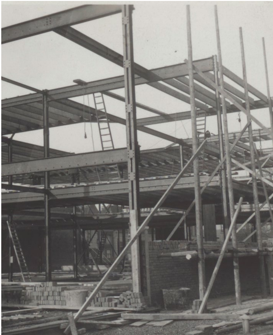
Photo: Bolted steel structure , from the historical report of Voorstraat 258(NIPIDES, 2020)
