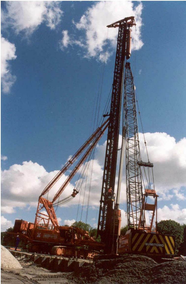
Figure 6 Pile driving: a very difficult source to describe
