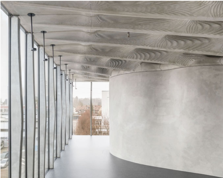
Fig. 2.16 Final installation of façade mullions in the DFAB House, on the left-hand side of the image
