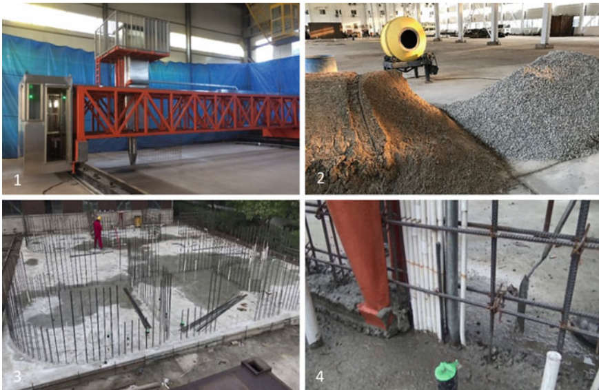
Fig. 2.23 On-site 3D-printing by HuaShang Tengda: 1. gantry-based printer with a hopper on the top of the printhead; 2. raw materials and mixer; 3. foundation and connective steel bars; 4. deposition of the first layer
