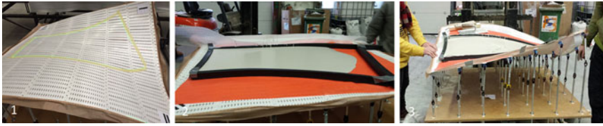
Fig. 2.20 Prototype of the flexible mould as developed in a Dutch R&D project operating in mode 1, deformation: Setting out formwork (Schipper et al. 2015b)
