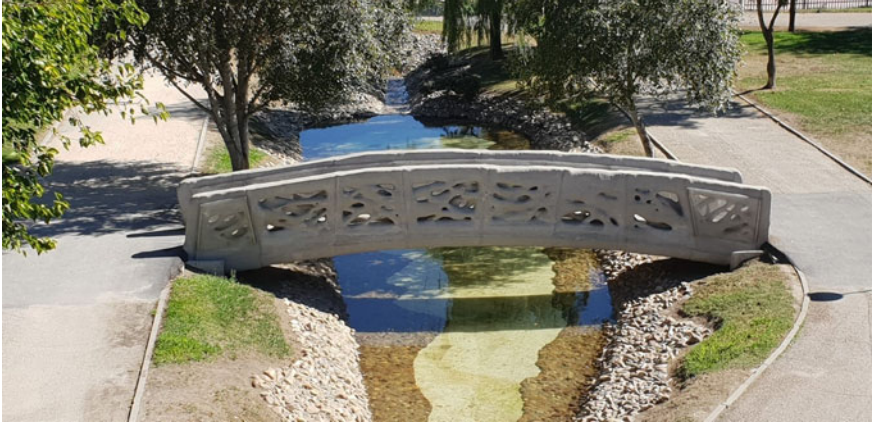
Fig. 2.13 The footpath bridge in Madrid by Acciona (© Enrico Dini)
