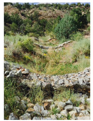
[Figure 141.] Example of gully rehabilitation by gabion checkdams (Doten, 2020)
