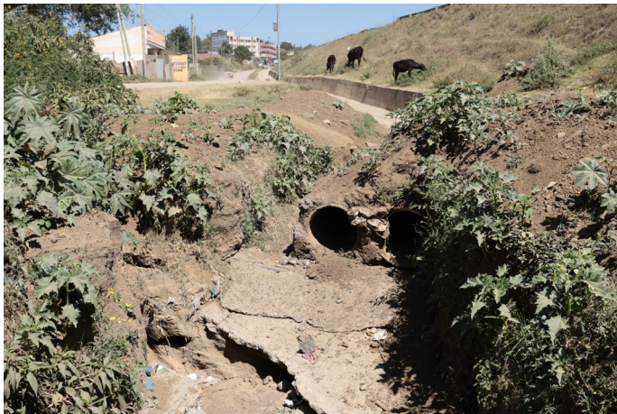
[Figure 168.] Erosion of conventional culvert (photo by author)
