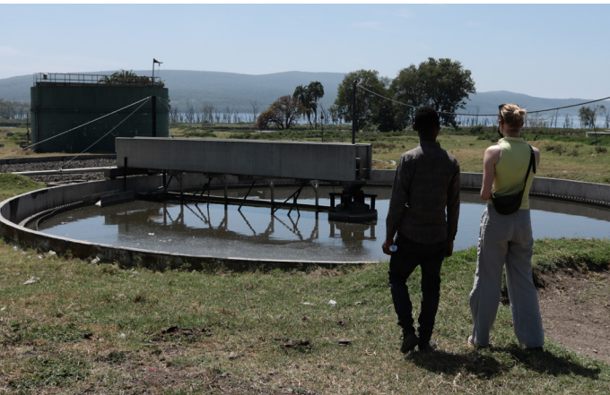
[Figure 165.] Machinal system for treatment of sewage was out of system, which led to severe pollution of the surroundings, especially of National Park Lake Nakuru in the background.
