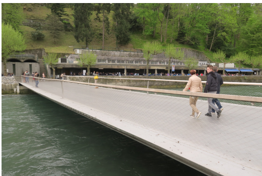
(a) Footbridge in Lourdes [16]
