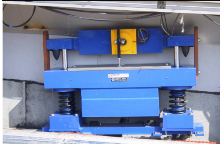
Figure 2.15: An example of an implemented TMD for vertical vibration mitigation [28]
