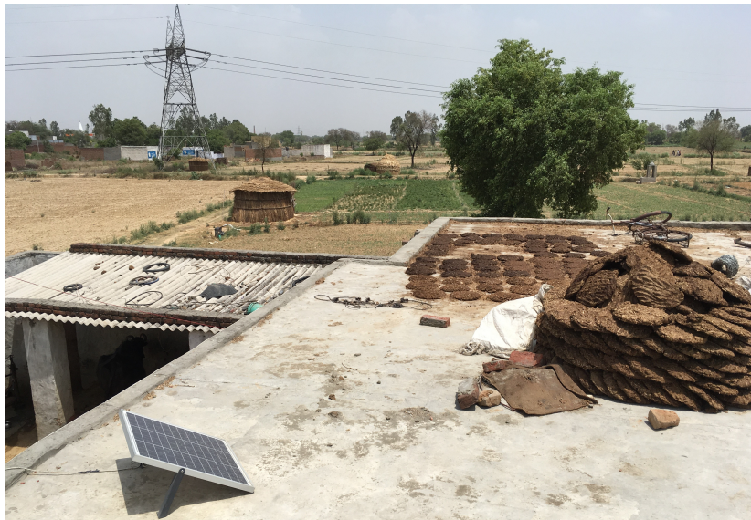
Figure 2. So close, yet so far: A rural household in Aligarh, Uttar Pradesh (India) with installed SHS. Grid lines have passed close to the house for years, yet the household was without any grid-based electricity until 2017. Photo credit: Gaurav Manchanda.
