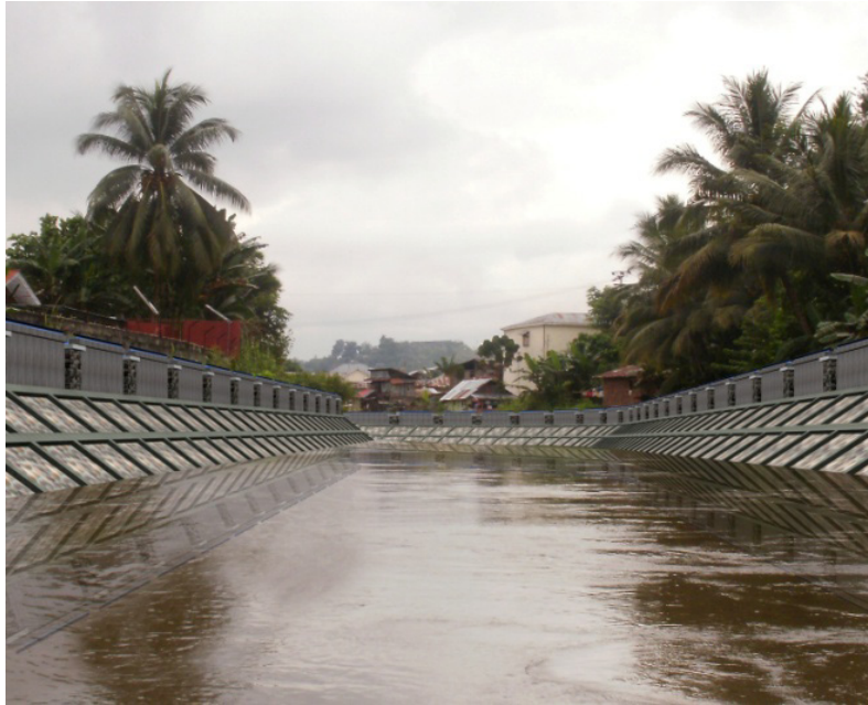
Figure 11: Artist Impression of Urban Flood Control plan, example of 'smoothing of bends
