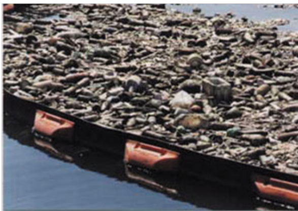
Figure 21: Floatable barrier to collect garbage
