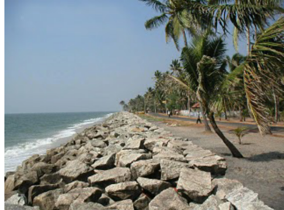
Figure 27: Rubble coastal protection
