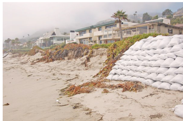
Figure 28: Coastal protection with sandbags
