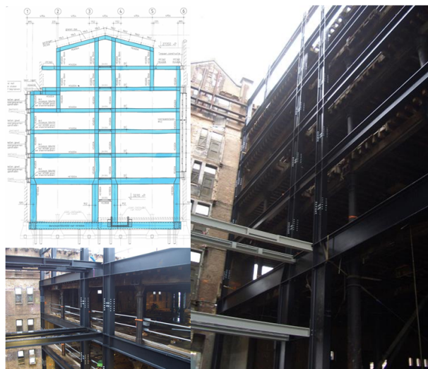
Figure 4-33 Jobsveem - Stabilizing system in the transverse direction
