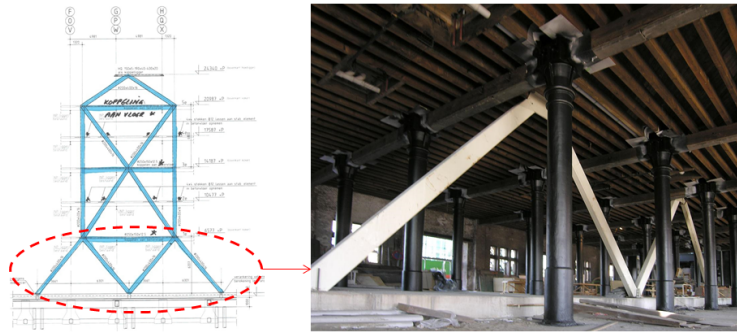
Figure 4-34 Jobsveem - Stabilizing system in the longitudinal direction
