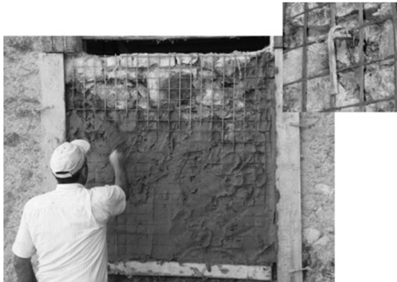
Figure 3-17 Application of mortar jacketing and detail of connection between anchors and GFRP grid (Corradi, Borri, Castori, & Sisti, 2014)
