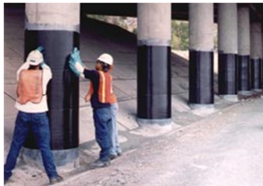
Figure 3-6 Applying FRP sheets on circular reinforced concrete columns.
