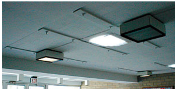
Figure 3-15 Roof slab strengthened with a combination of FRP and steel plates.
