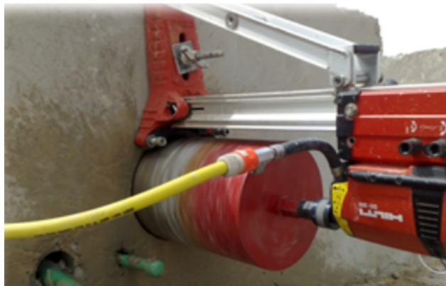
Figure 3-2 Concrete core cutting (Skill Gulf, 2015)
