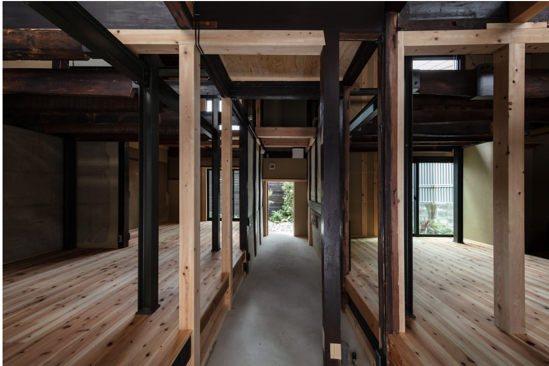
Figure 8: Container House Structures (Sasakura, 2020)
