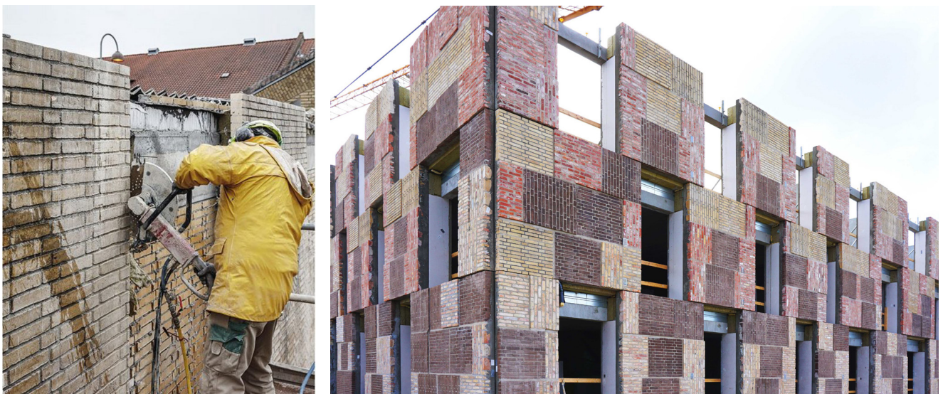
Figure 81 - Resource Row Project by Lendager Group; (left) brick elements cut from building, and (right) upcycled brick wall in the building (source: https://lendager.com/en/architecture/resource-rows/#materials )
