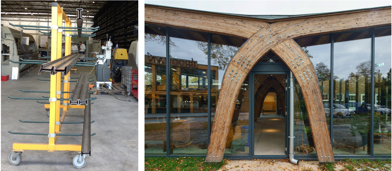
Figure 82 - KEVN Pavilion Eindhoven by Superuse Studios; (left) steel profiles from construction overstock, and (right) reused steel profiles in the pavilion clicked by Frans Hanswijk (source: ODS)
