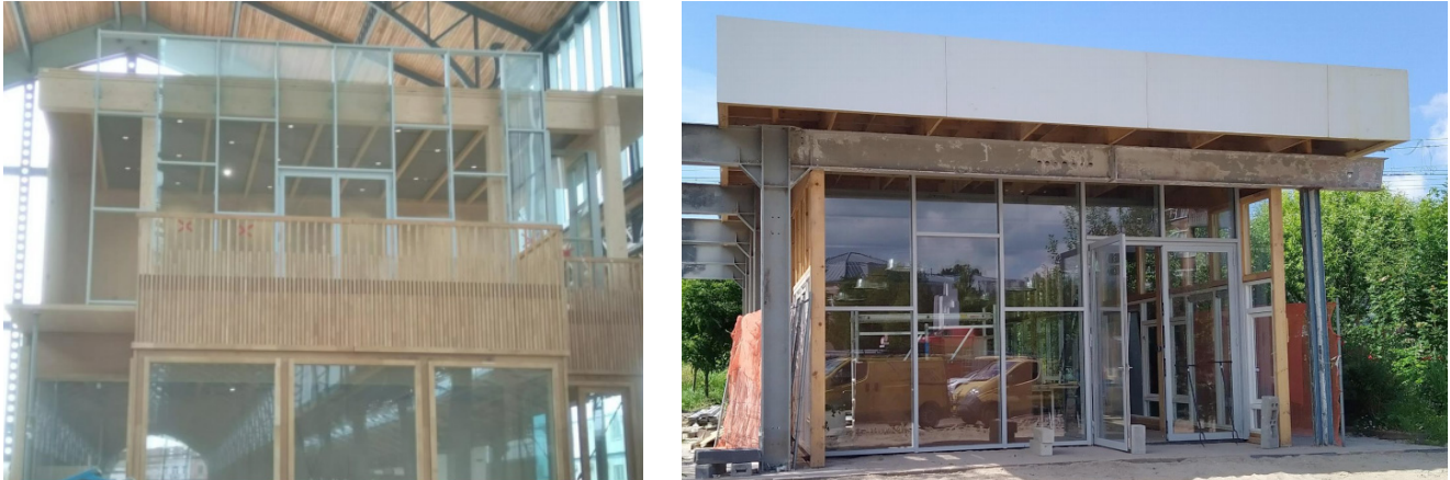
Figure 33 - (left) Mockup facade for Gare Maritime, Brussels, and (right) Reused façade for The Field, Leiden (source: Harvest Bay Platform)
