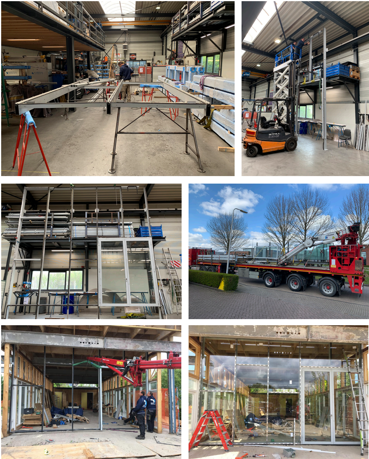
Figure 34 - Remanufacturing of the facade at the Blonkstaal Factory and installation on site (source: Blonkstaal Facade Builder)
