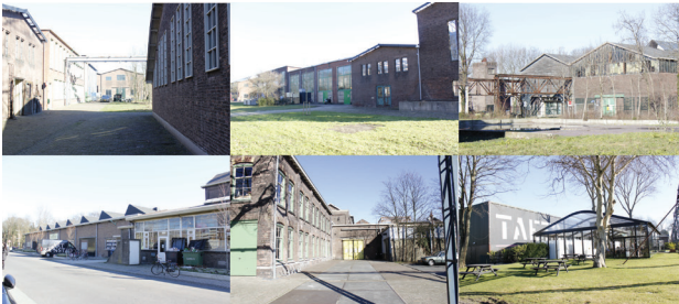
fig-73: the first 5 images (anticlockwise) show the repetitive architecture, the last image on the bottom right shows a contrasting piece of architecture on the same site
