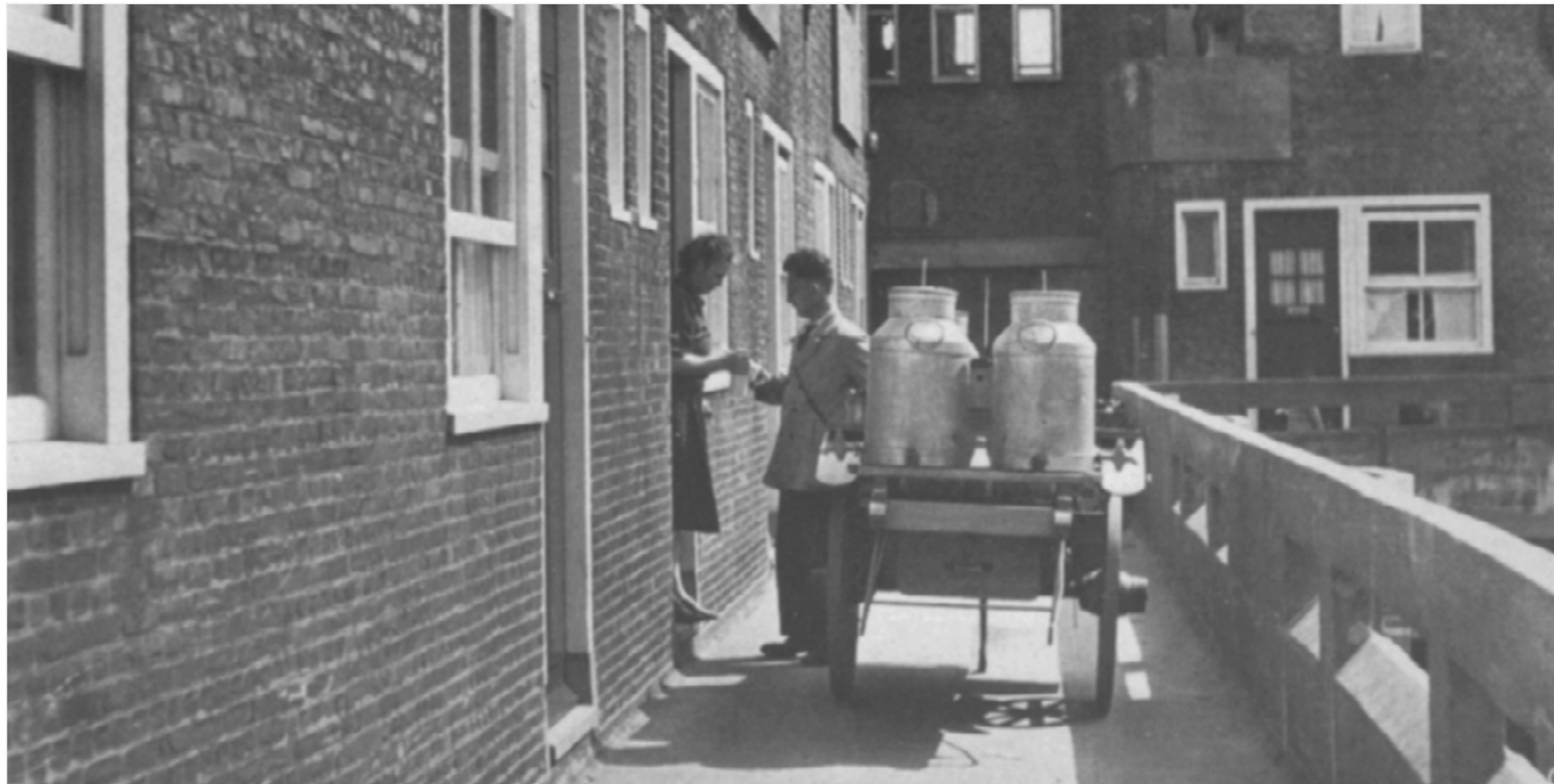
JUSTUS VAN EFFENCOMPLEX, ROTTERDAM
