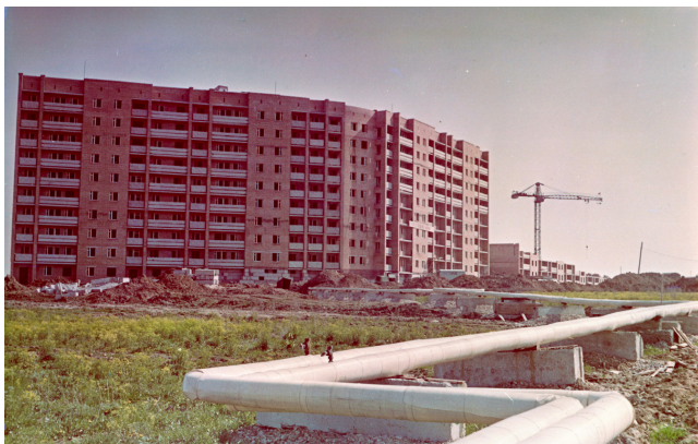
Figure 10. Pravoberezhny district under construction, 1987-1988, using a tetrahedral grid out of block-sections to shielded the inner-courtyard of the block from the prevailing wind [27].
