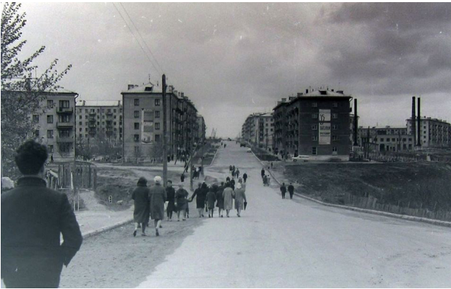
Figure 4. Photo of micro-district Cheryomushki few years after its completion, 1966 [27]
