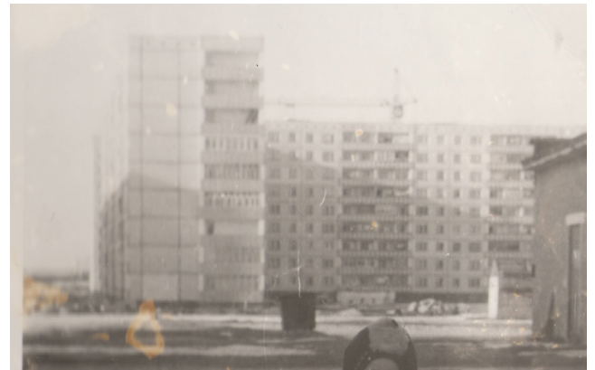
Figure 11. micro-district Kubyaka under construction, 1990 [27]
