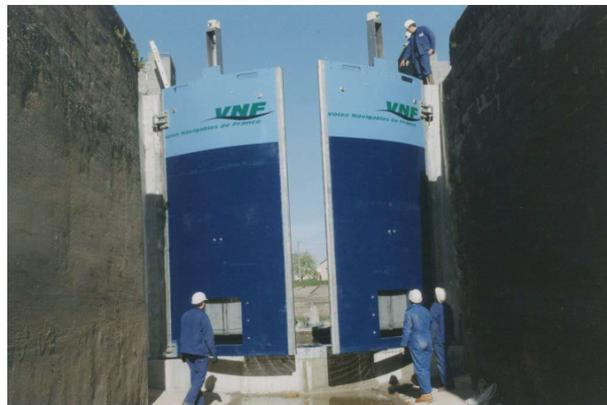
Figure D.1: GFRP gate lock Golbey PIANC (2009)
