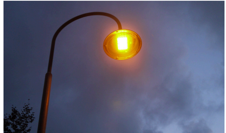
Figure 3.23. An example of a batlamp. Light is soft and warm and has no negative effect on bats, insects and other nocturnal animals (Hommen, 2022)
