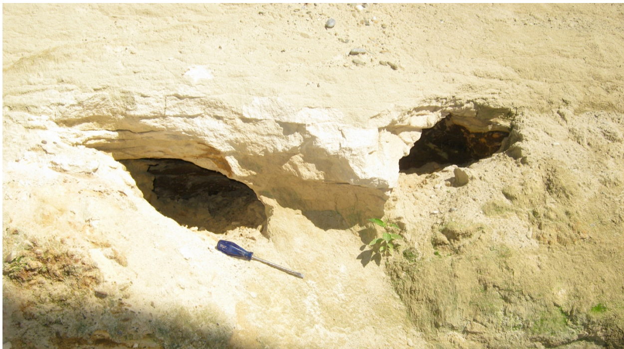
Figure 6: Karst phenomena visible at the A2 tunnel construction site [personal photograph, 2013].
