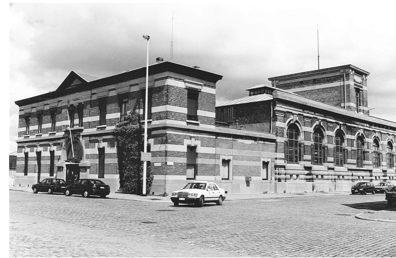
New machine hall and Site Entrance removal Later New Electricity Station
