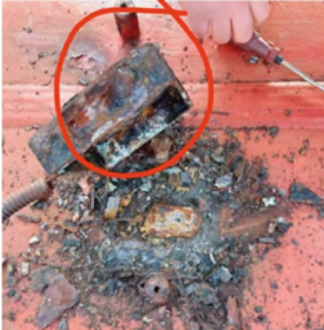
Fig. 1. Corrosion of optical fiber strain gauges of a SHM system
