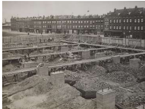
Picture F.16 The Foundation
