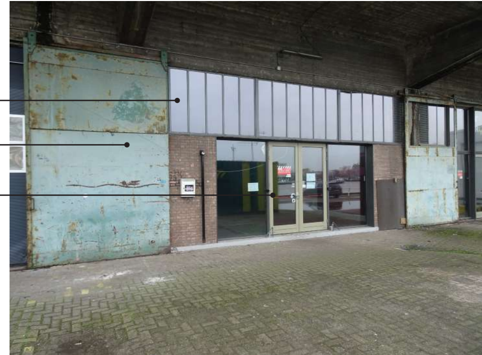
Picture M.50 - Close-up of the facade on the quayside
