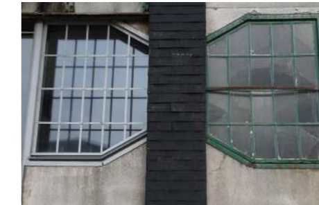
Picture F.30 - Windows
