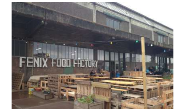
2013 empty terrace on the water side
