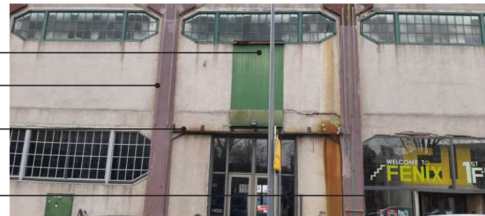
Picture M.51 - Close-up of a facade on the Streetside, (M. Bos, 2020)
