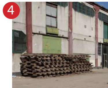
picture G.16 Current situation of railway
