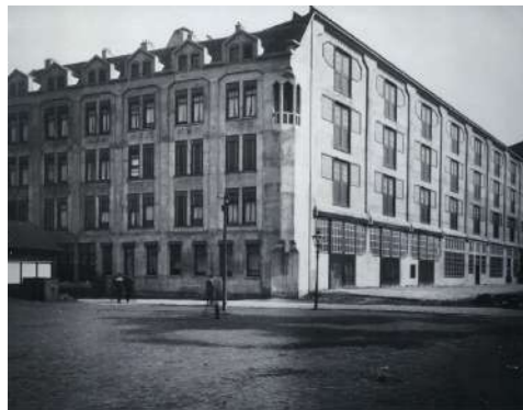
San Francisco Loods, Rotterdam 1922
