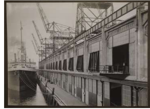
Picture M.52 - The bridges quayside In this picture it is visible how the bidge works (open)
