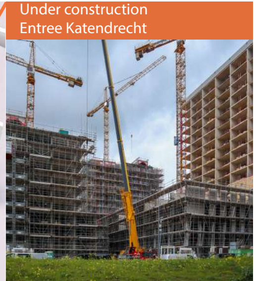
Picture G.12 Entree Katendrecht Current situation under construction.
