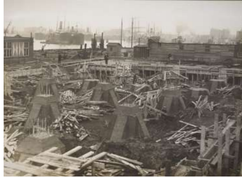
Picture F.15 The Foundation
