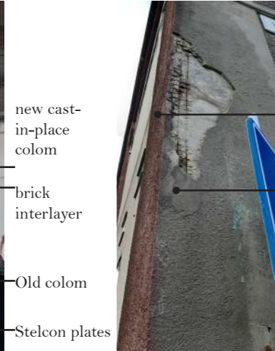
Picture M.45 - Close-up of colom at the corner.
