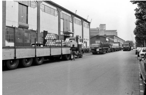
1950's the building on the road side
