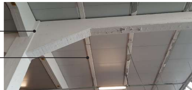
Picture M.48 - First floor
