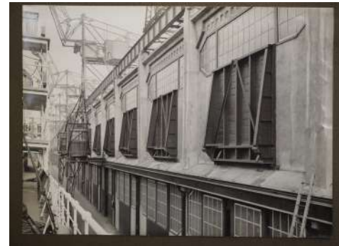
Picture M.53 - The bridge quayside closed it is visible that cranes move along the quay when the bridges are closed.
