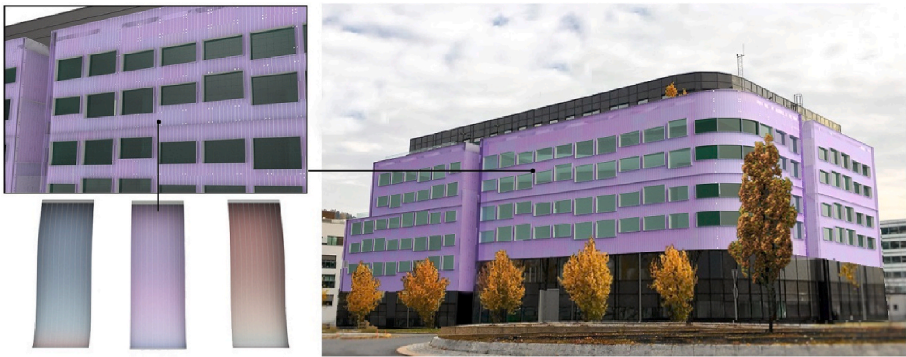
Fig. 3. Solsmaragden building skin with the PSC envelope.
