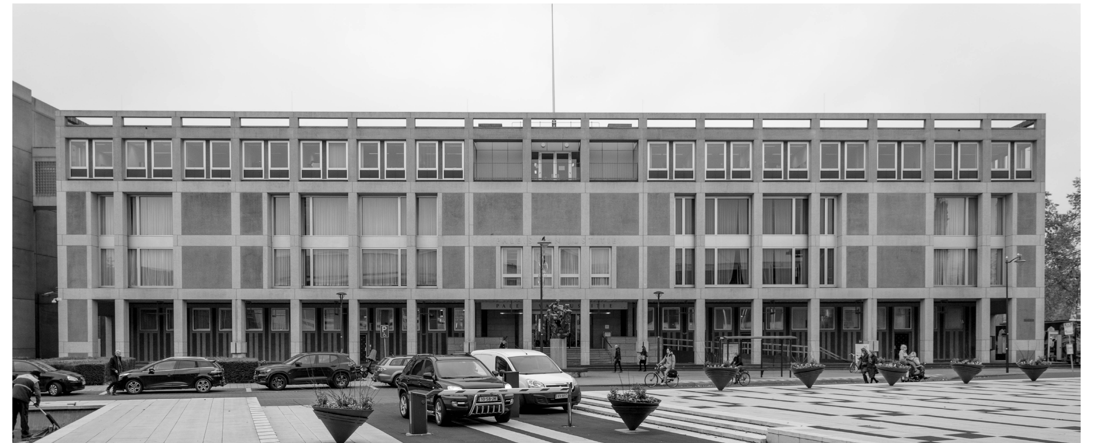
Main building Completed : 1963 Architect: F. Sevenhuijsen
