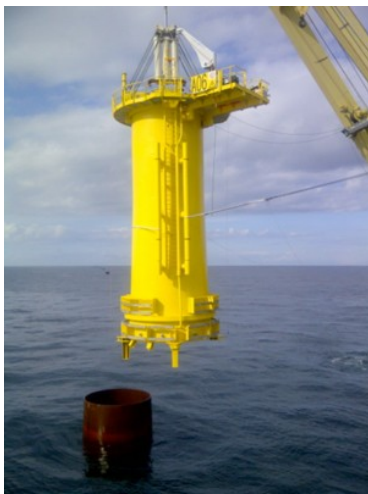
(a) Lifting of the transition piece at Anholt wind farm [W2]
