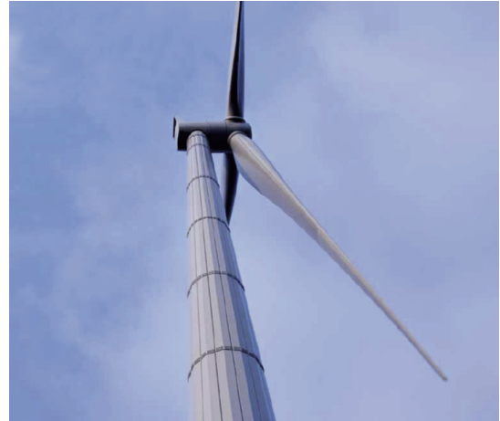
(b) Steel shell tower concept [W29]
