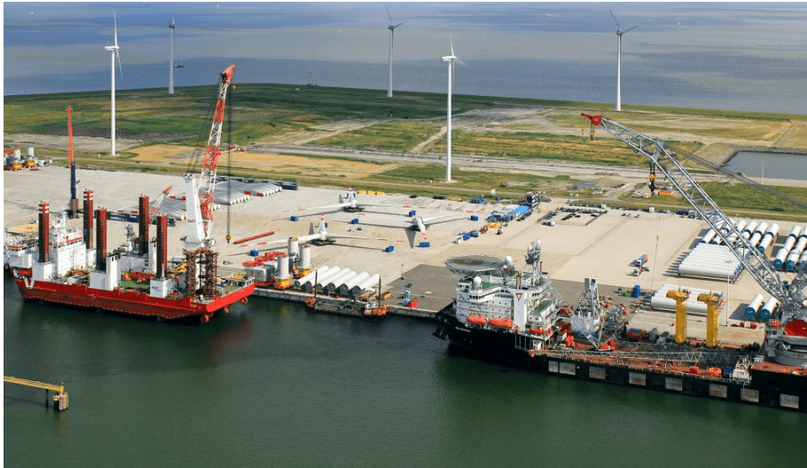
Figure 3.4: Onshore assembling of the turbine at Eemshaven [W5]
