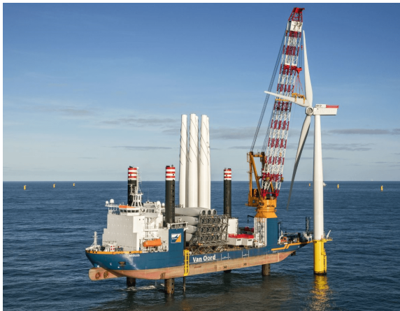
(a) Jack up vessel at Gemini wind farm [W21]
