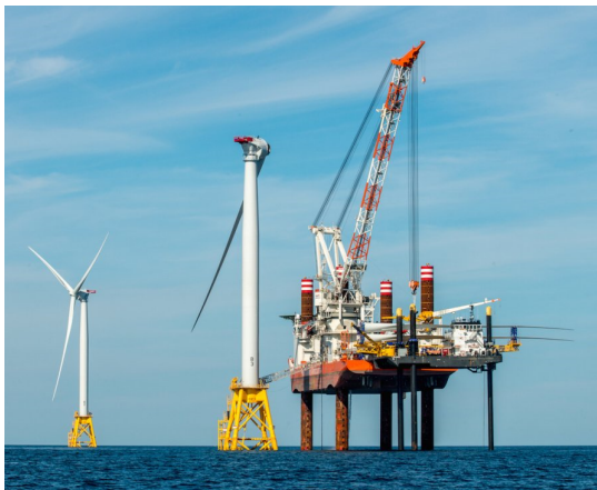
(a) Installation of blades at a US wind farm [W8]
