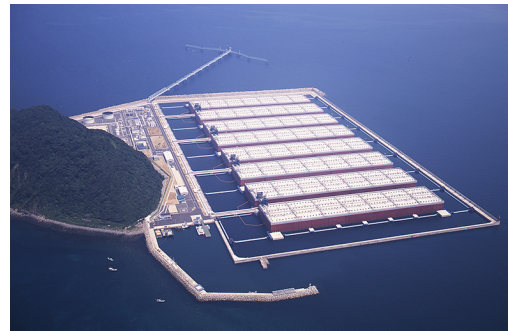
(b) Oil storage base at Kamigoto Island [201]
