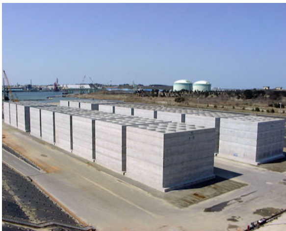
(a) Construction of caissons [W16]
