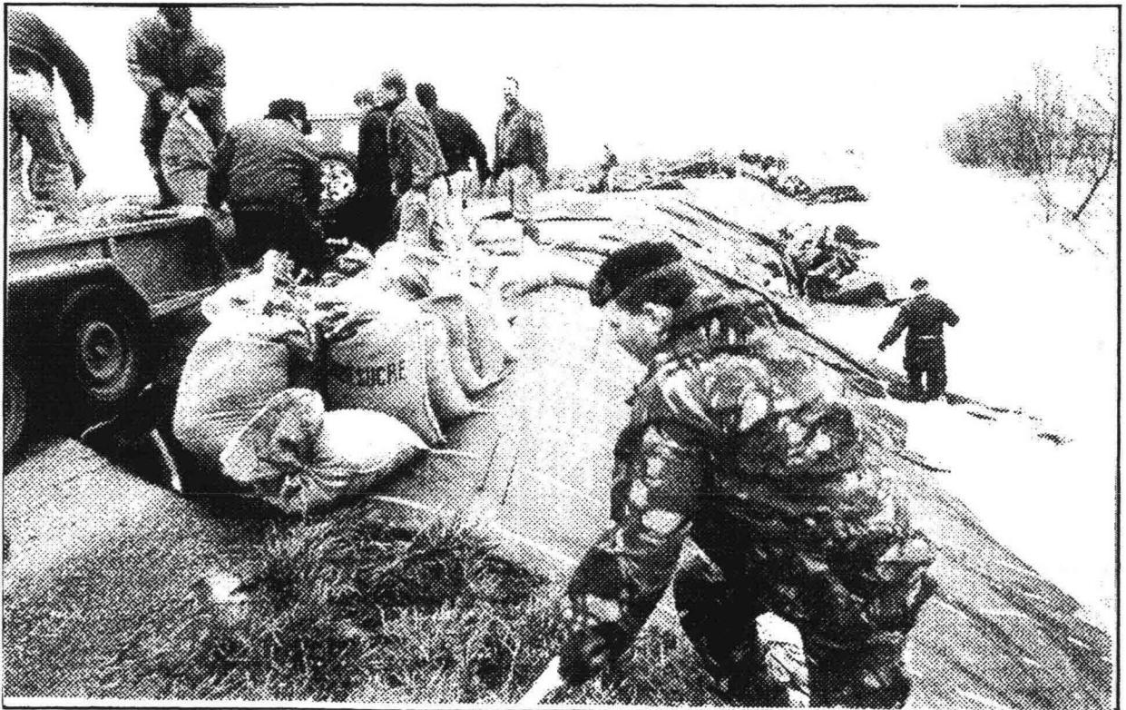
Figure 11.7: Geotextile used to protect a grass slope
