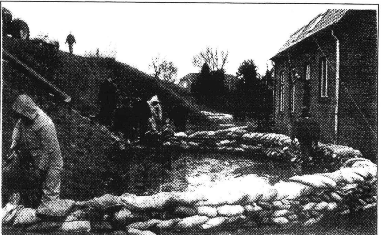
Figure 11.4: Emergency wall of sandbags around a well
