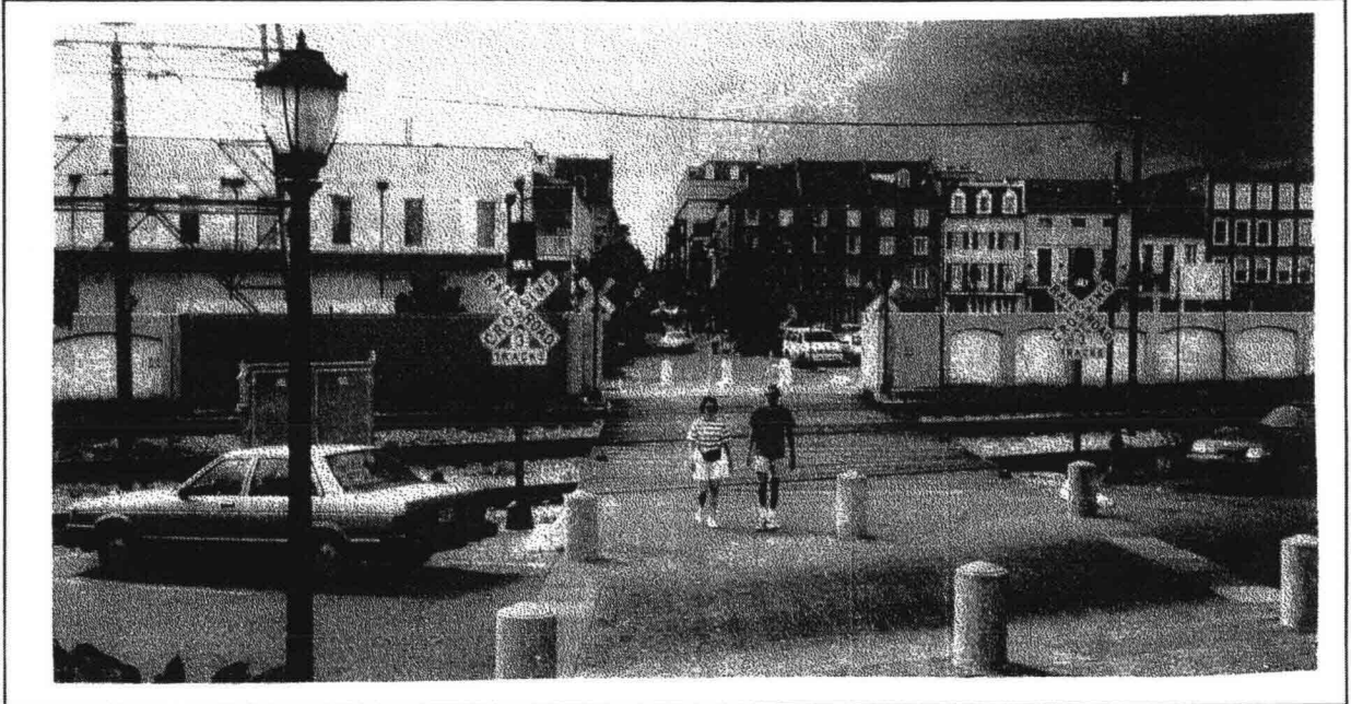
Figure 11.1: Gap in a streetcar crossing in the river-levees of New Orleans
